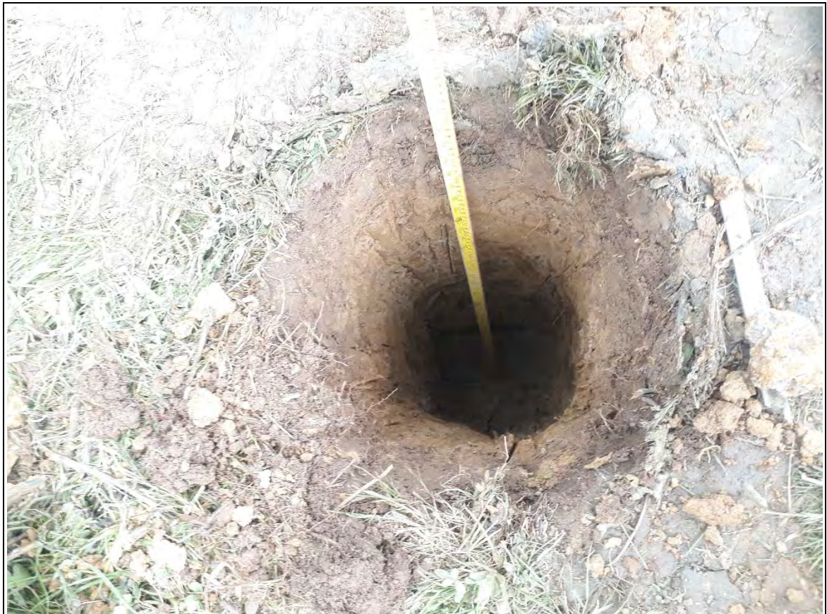
Borehole: CP104A Inspection pit
